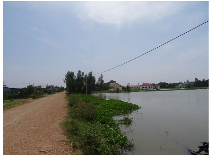
Climate-resilient road in Borei Chulsar Commune, Takeo
