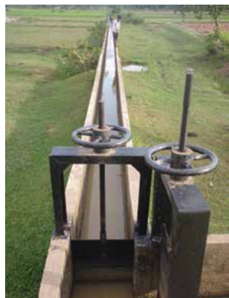
Concrete canals at O Krasar, Kep province
