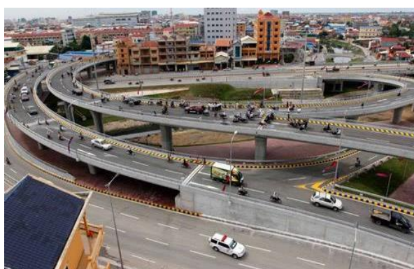
Photo 33: Sky-bridge construction to reduce traffic congestion and road accident (Source: MoE)
