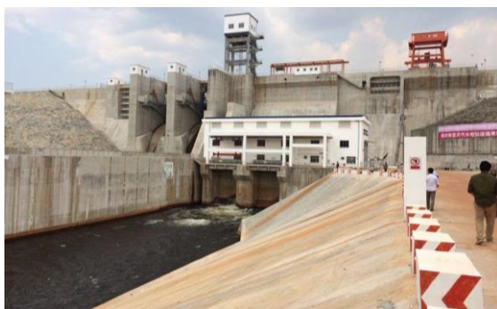
Photo 23: Hydropower construction for power generation (Source: MoE)
