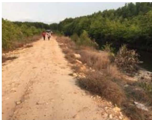
Banks of a sea dyke are planted with grass and small mangrove plants for slope protection.
