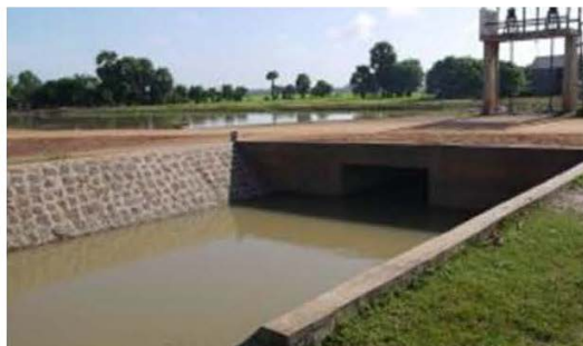
Culvert and sluce gate in the rehabilitated tributary canal of the Prasat system in Kampong Thom Province (pictured on 7th October 2015)
