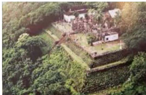
Bank slope protection at Phnom Chiso Temple (Takeo province, CAMBODIA), 11th century.
