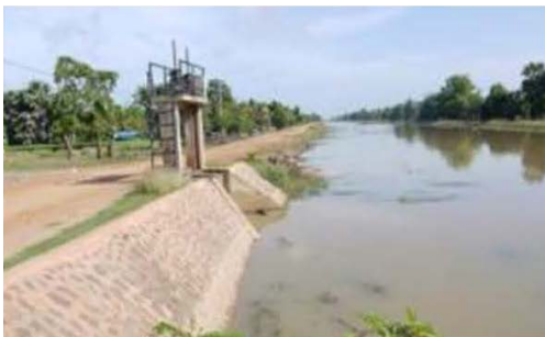
Main canal of Samseb-Kanha Dam in the Prasat irrigation system in Kampong Thom Province, rehabilitated and renovated by ADB project (pictured on 7th October 2015)
