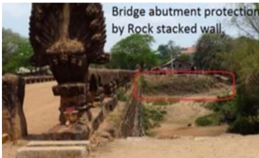
Bridge abutment protection by Rock stacked wall at Kampong Kdei Bridge (Siem Reap, CAMBODIA), 12th century.
