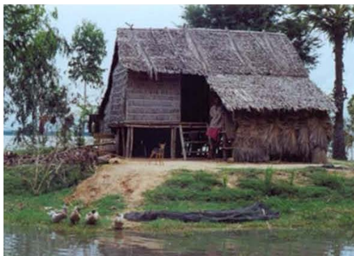
Safety hills providing refuge from flooding for a single house
