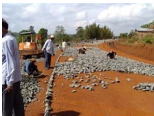
Macadam base course works: the stone to be laid by hand (source: Monduliri's DPWT)
