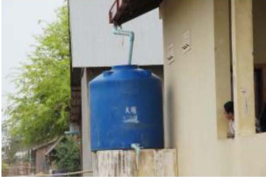
A roof rainwater collection system of Sre Houy community in Sre Houy village, Sre Houy commune, Koh Nhek district, Mondulkiri province.
