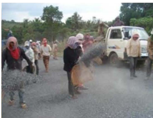
Macadam base course works: the aggregate to be laid by hand (source: Monduliri's DPWT)
