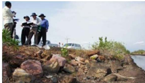
Amour rock used to protect bank erosion
