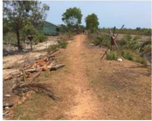
The dyke protects farmland from saltwater.
