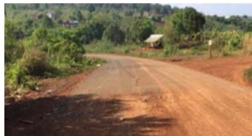
DPWT upgraded the Laterite road built by MRD to macadam base DBST pavement (section in town)
