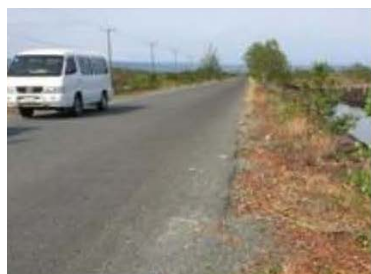
Macadam road in Koh Kong (finished 2013), Photo: April 2016. It passed through two monsoon seasons and the pavement is in good condition.
