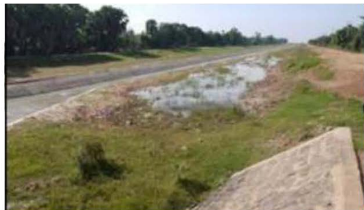
The concrete canal in the main canal of Samseb-Kanha Dam in the Prasat irrigation system in Kampong Thom Province, rehabilitated and renovated by a China-funded project (pictured on 7th October 2015)
