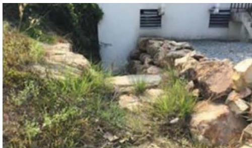
Stone wall as a storm water drain (Tatai Bridge, Koh Kong), Photo: April 2016
