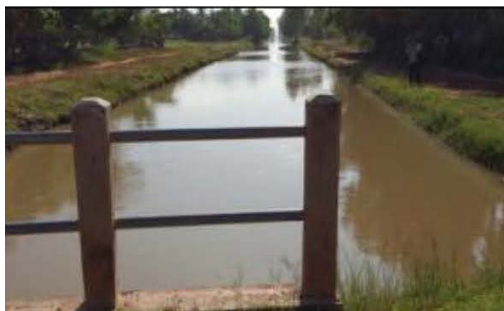
Tributary canal (Samdach Techo Canal) of Prasat system in Kampong Thom Province, rehabilitated by Military Engineering Forces in 2008 (pictured on 7th October 2015)
