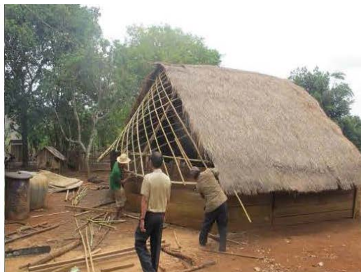
Construction of houses using bamboo and thatch
