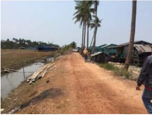
Sea dyke in Chimeal village, Andoung Toek Commune, Botum Sakor district. It is used to prevent seawater intrusion into farmland.
