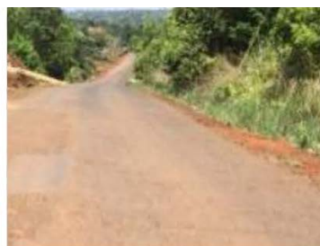
Macadam road in Monduliri (finished-2004), Photo: April 2016. It passed through 12 monsoon seasons and the pavement is in good condition.
