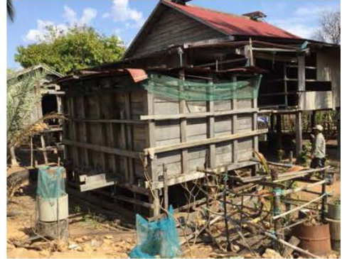
A roof rainwater collection system with a typical wooden tank, Norng Bour village, Norng Khiloeok commune, Koh Nhek district, Mondulkiri province. It was built in 2012 by the residing family.
