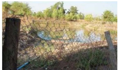
Excavated pond fenced by wire-net is in Mean Chhey village, Sre Sangkum commune, Koh Nhek district, built in 2010-2011 by the Provincial Department of Rural Development, and managed by a water user community.
