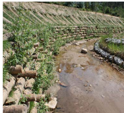
Gully treatment using live crib wall
