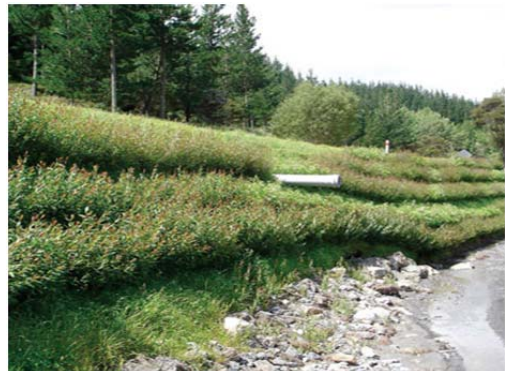
Live staking to control erosion in New Zealand
