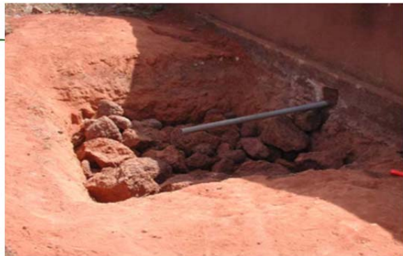
Soak pit with installed PVC pipes
