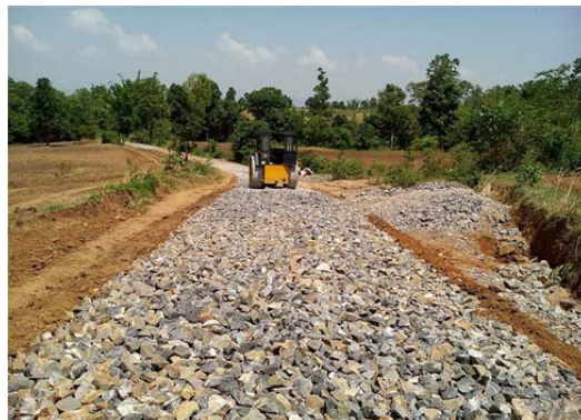
Macadam road in Cambodia
