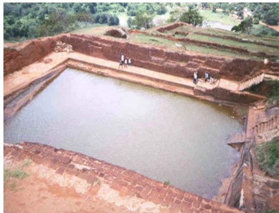
Rainwater harvesting pond in Sigiriya, Sri Lanka
