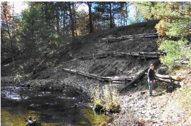
Log terracing prevent sand from sliding down the bank
