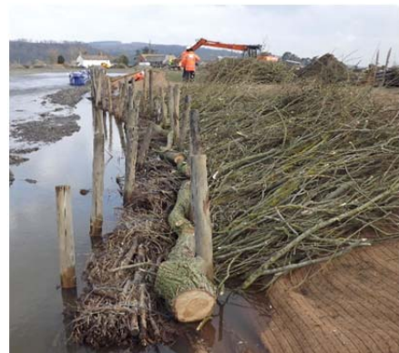
Installing vegetated revetment
