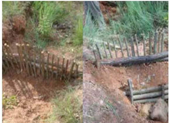
Palisades stabilise gully floor and trap material
