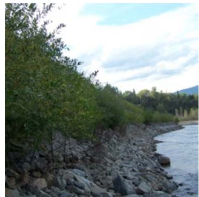
Vegetated riprap along a riverbank
