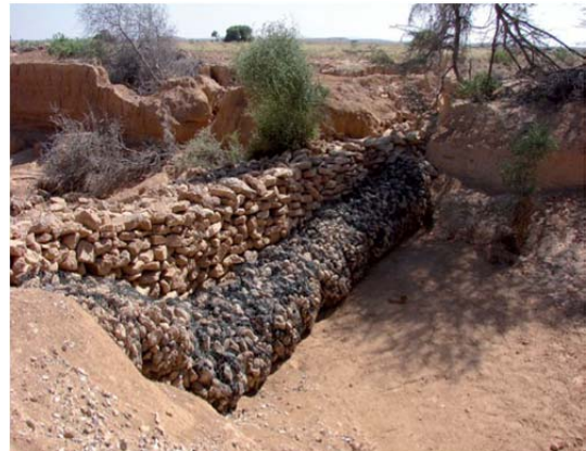
Check dam stopping gully erosion in East Africa
