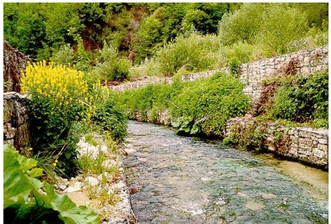
Example of vegetated gabion channel
