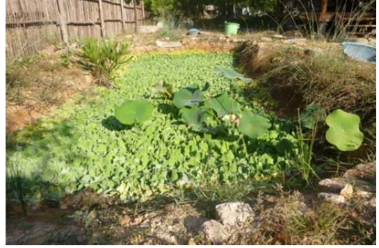
Polishing pond for single family treatment in Sihanoukville, Cambodia
