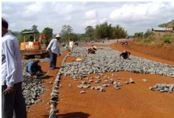
Building a macadam road in Cambodia
