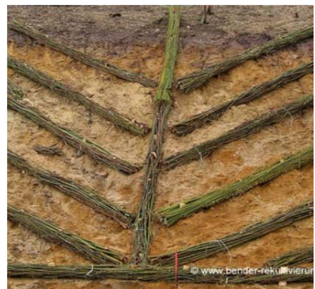
Live fascine protects slope from erosion
