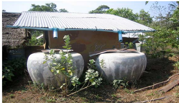
Illustration of a rainwater harvesting system
