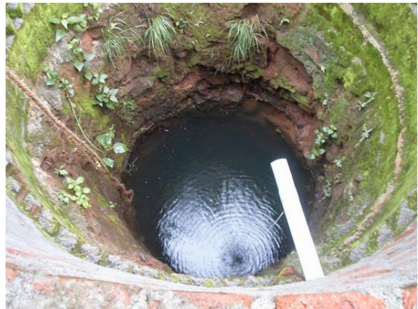
Recharge pit with plenty of water
