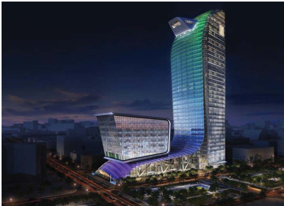
Figure 12. Energy Efficient Building in Phnom Penh
