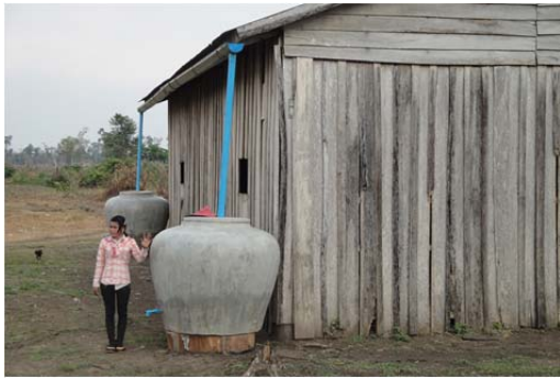
Typical rainwater catchment system
