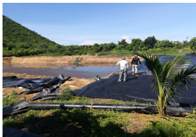
INSTALLATION OF COVERED LAGOON AT ONE OF THE SELECTED FARMS
