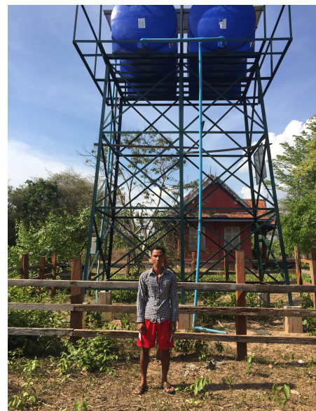
Than in front of the batch tank that connects the pump and the main pipe.
