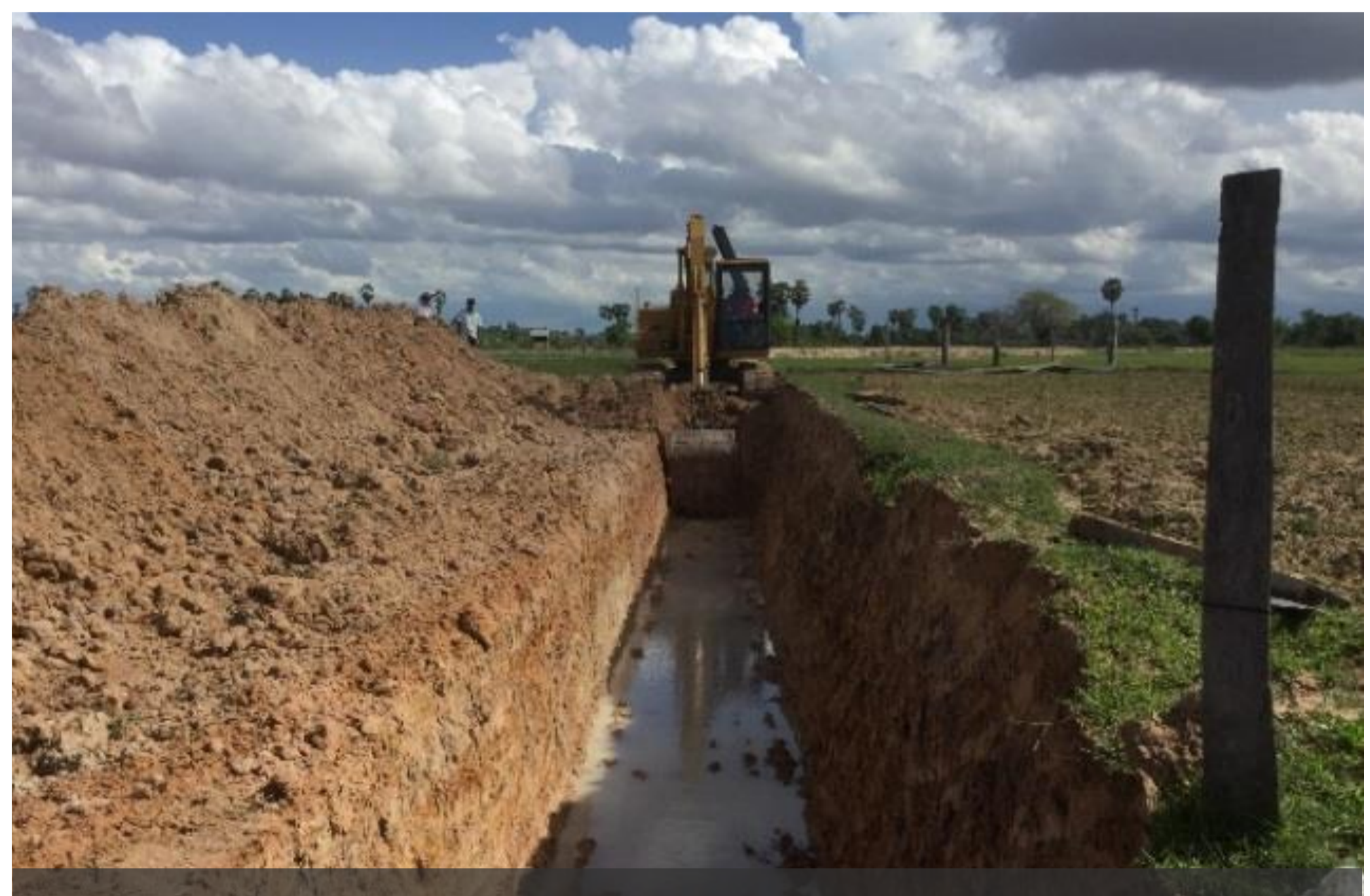
Irrigation system rehabilitation in Trapeang Chan commune, Kampong Chhnang
