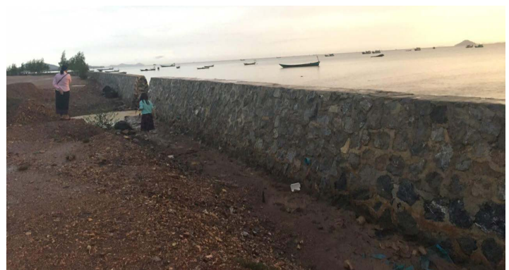
Sea wall along the seashore to prevent salt intrusion
