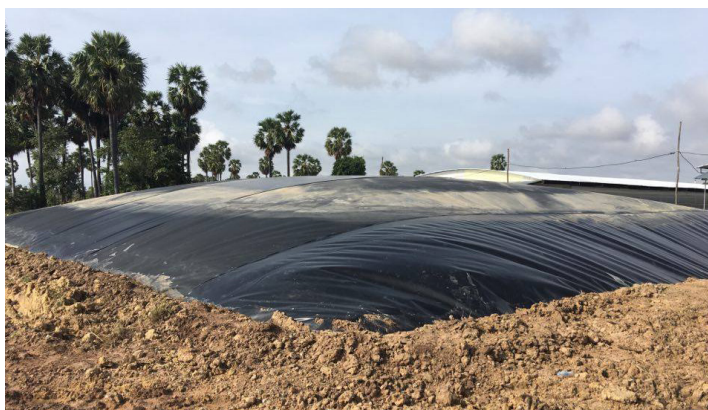
Medium scale biodigester dome storing pig dung in Kampong Speu's Kong Pisey district, in December 2016
