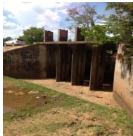
Khsaet Lake existing embankment and sluice gates
