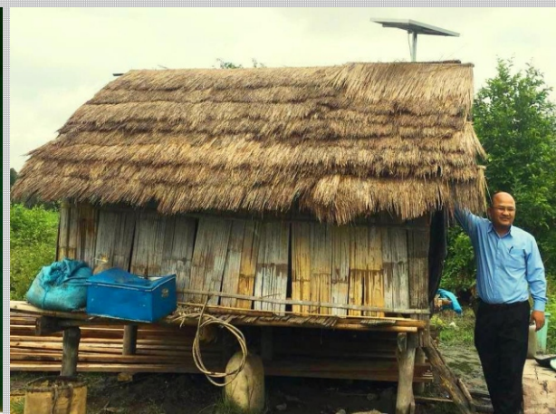
Solar electric system is equipped to villagers of target CFs, MKR
