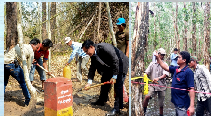
CPA pole-installation CPA Management
