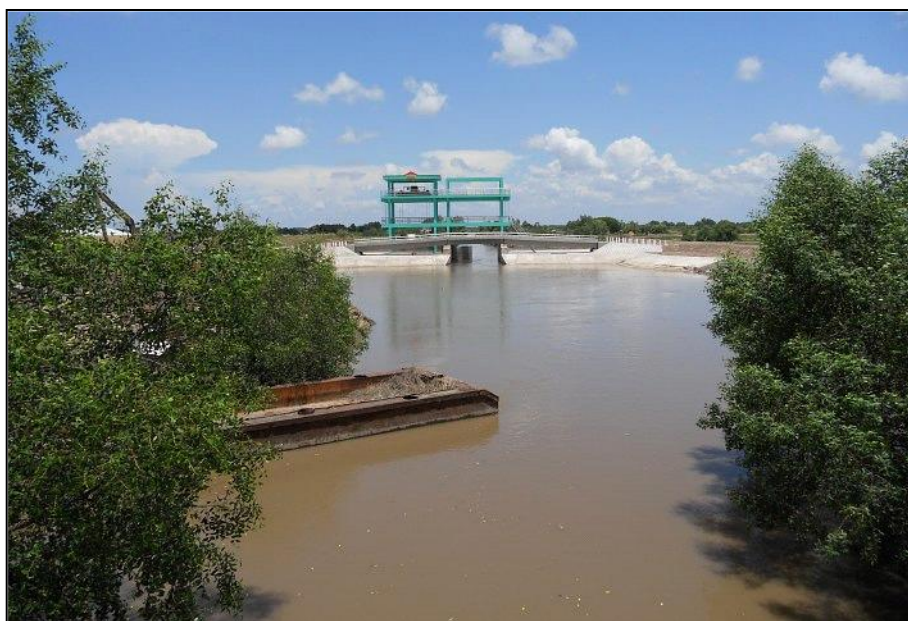
Figure B.10: A multi-purpose flow regulator, controlling inflows and outflows
