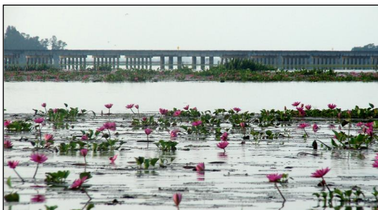
Figure B.8: The Thale Noi elevated causeway
