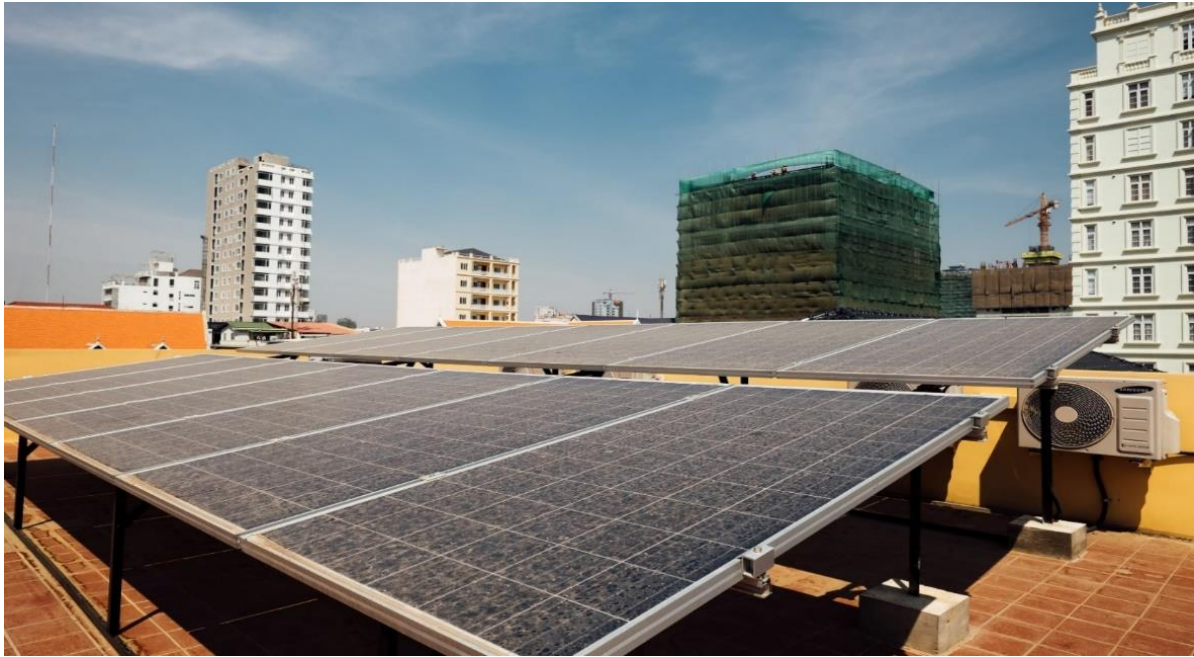
Figure 8. There is substantial potential for roof-top solar PV in Phnom Penh to service households, businesses and manufacturing (photograph by Bernardo Salce).
