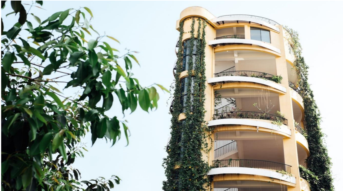
Figure 11. Green building design is already evident in some building in Phnom Penh. It enables electricity savings through the use of natural cooling systems (photograph by Bernardo Salce).
